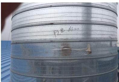
图5.排气筒P2监测孔
